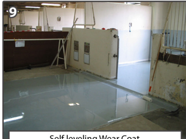
Self leveling Wear Coat applied
