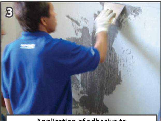
Application of adhesive to walls and floor
