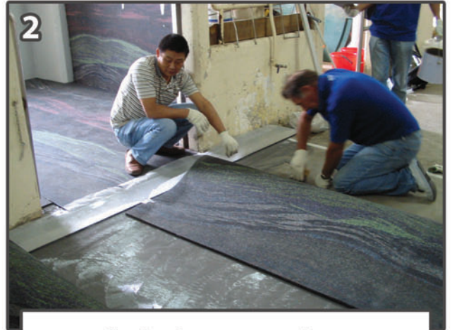
Cutting base mat to size
