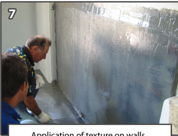
Application of texture on walls
