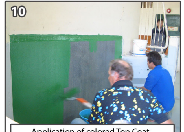
Application of colored Top Coat on walls
