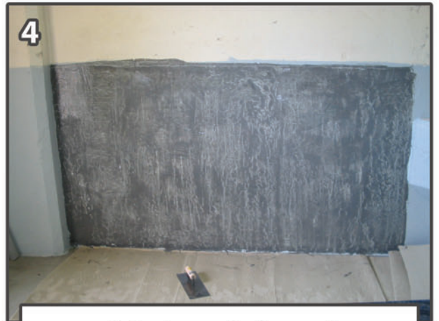
Adhesive applied on wall
